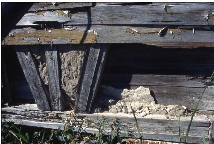
Image: Babin Place main house heavy timber-framed construction with mortise-and-tenon joinery secured with wooden pegs, bousillage walls, and cypress siding.
