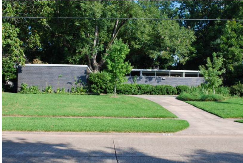
Photo 17. A classic soft modern house in Shreveport (architect unknown). The house totally turns its back to the street. The architect lifted the roof above the brick wall to create high windows.
